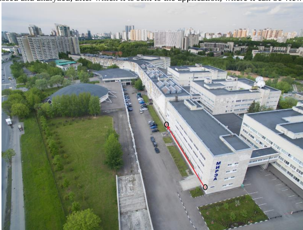
Fig. 1 Location of the transmitter and receiver of the strain monitoring system
